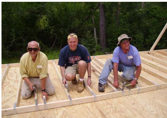
Mike Kendro & Clay Poindexter join Larry Mock assemble a wall.
